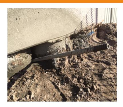
The anchor used is a 35mm Galvanised hollow bar, supplied in 3m lengths, installed to a length of 12m. Using a very low viscosity grout acting as a drilling fluid each hole took 35-40 minutes to drill. Prior to insertion of the third rod, the grouting operator utilised the second tank on the ChemGrout CG500HP to switch mixes to a higher density 0.45 brew.
